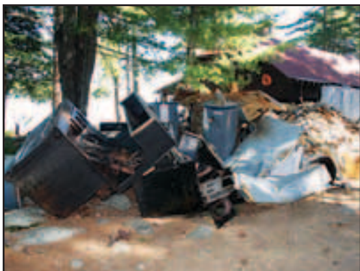
Camp Lawrence's kitchen project began with major demolition work which started right after the campers left this summer.
